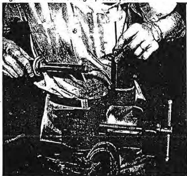
Fig. 3-5. Fillet welding a plastic joint.
