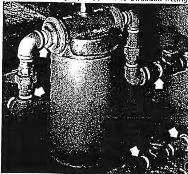
Fig. 6-9. Sealing tape applied to threaded fittings.
