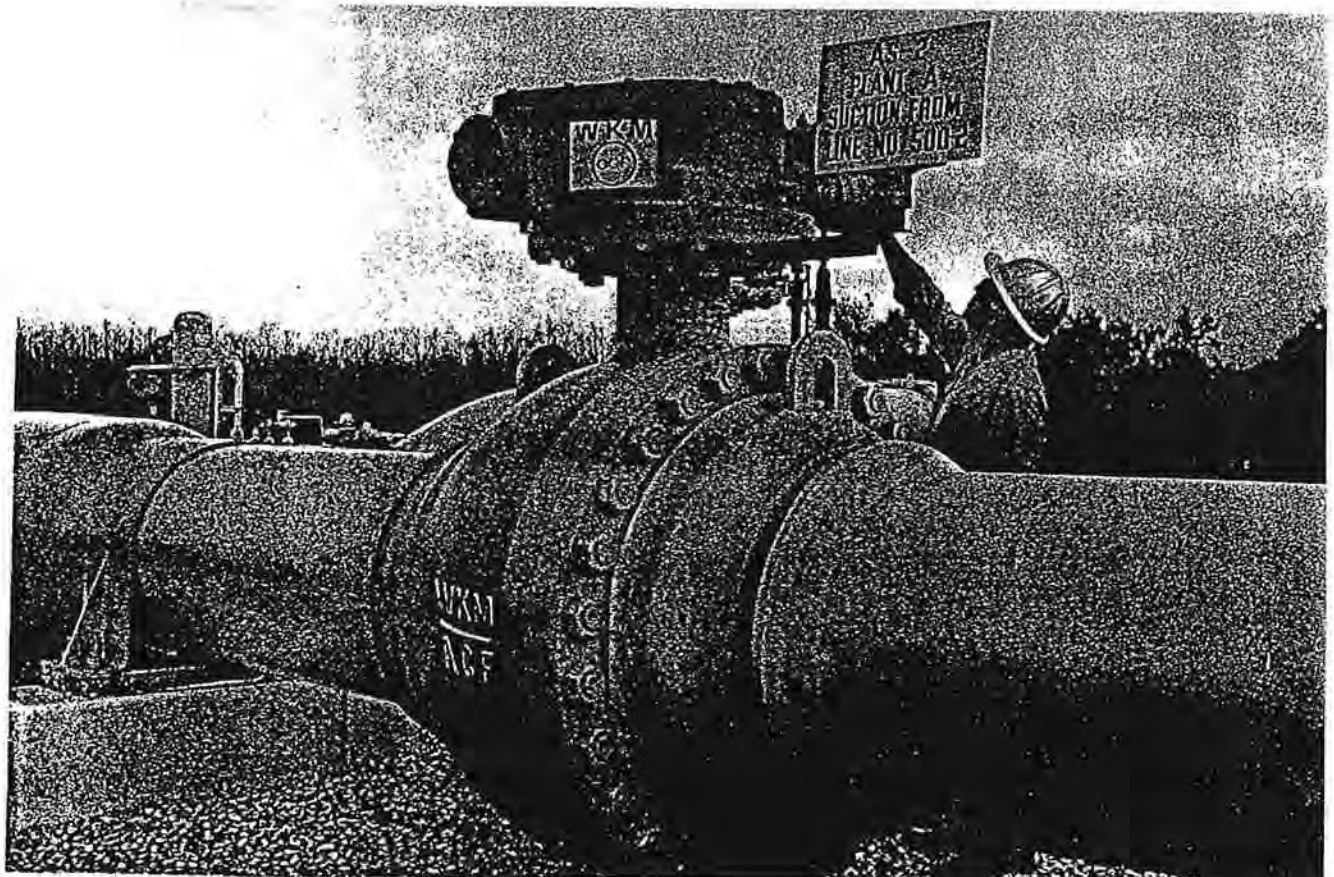
Fig. 8-15. Ball valve installation with mechanical actuator.
