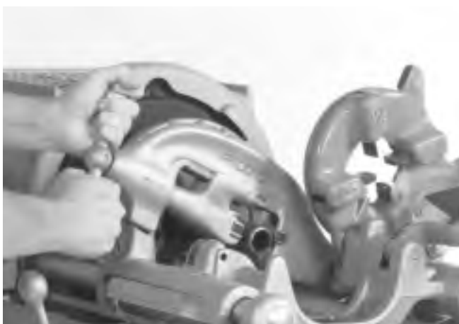
Figure 6 – Cutting Pipe with 820 Cutter
